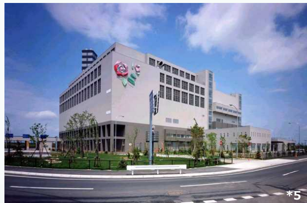
Waste treatment plant
